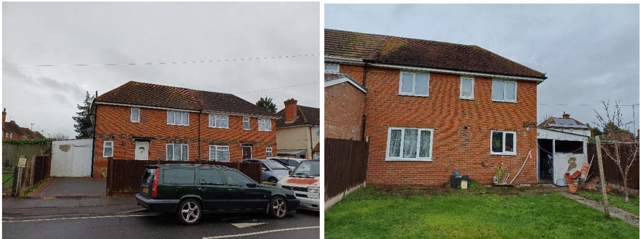
Figures 1 & 2: Views from the front and rear of 62 Stockton Road (12/01/2026)
