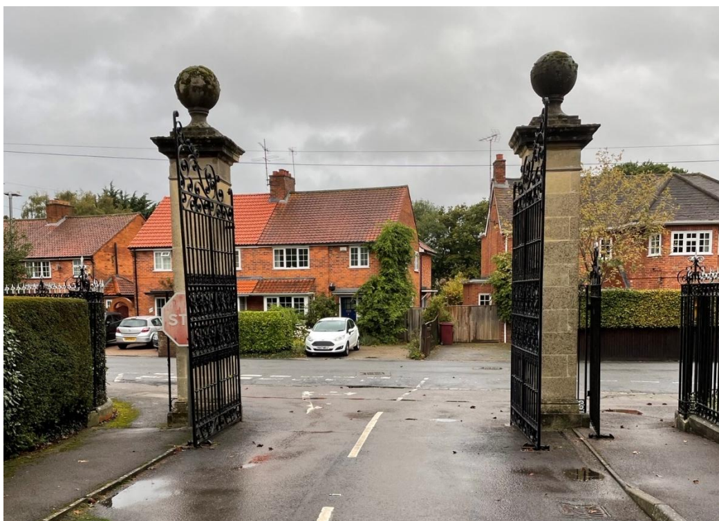
Both piers - rear
