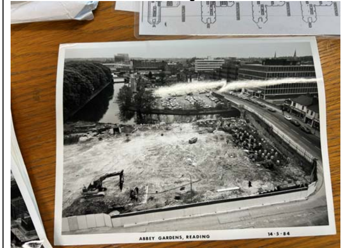
Photo 9: Site During Construction
