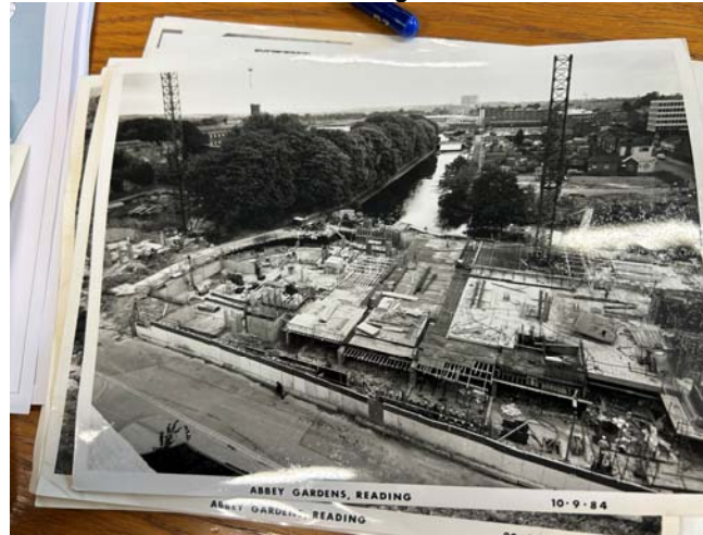
Photo 8: Site During Construction
