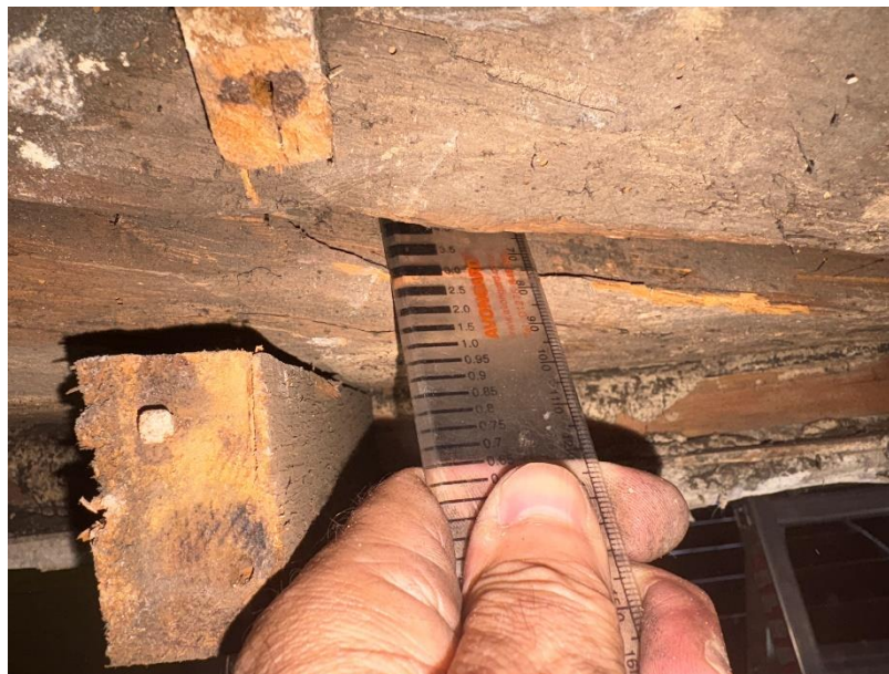
Figure 13. Split depth in valley beam width.
