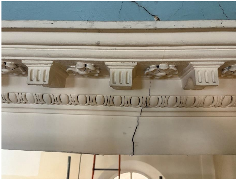
Figure 10. Valley beam prior to intrusive inspection.
