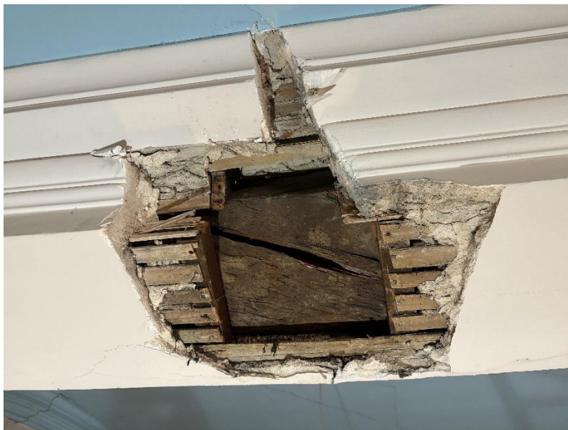
Figure 11. Valley beam after intrusive inspection.
