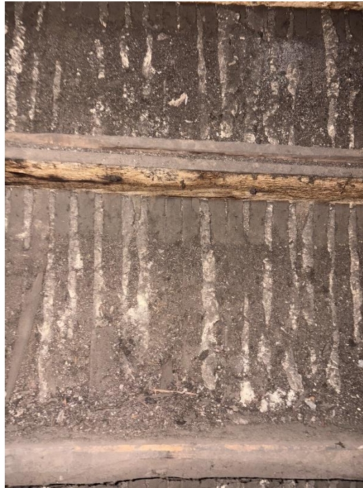
Figure 6. Lath and plaster ceiling construction from within roof void.
