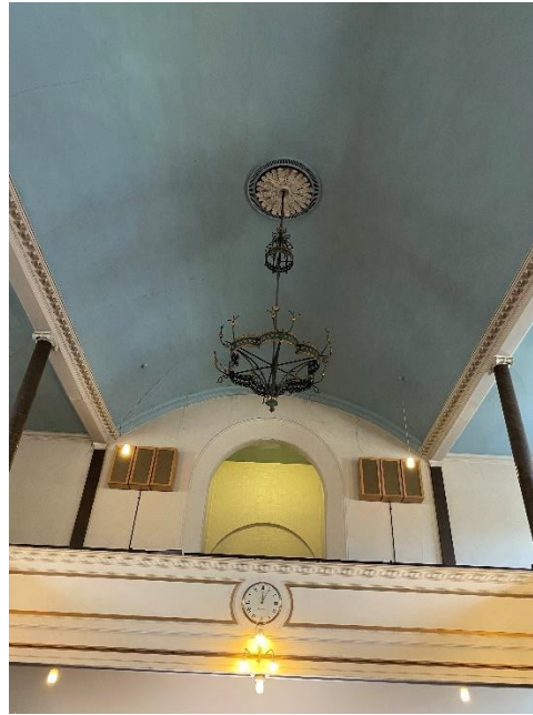
Figure 4. Ceiling to the south end of the church.
