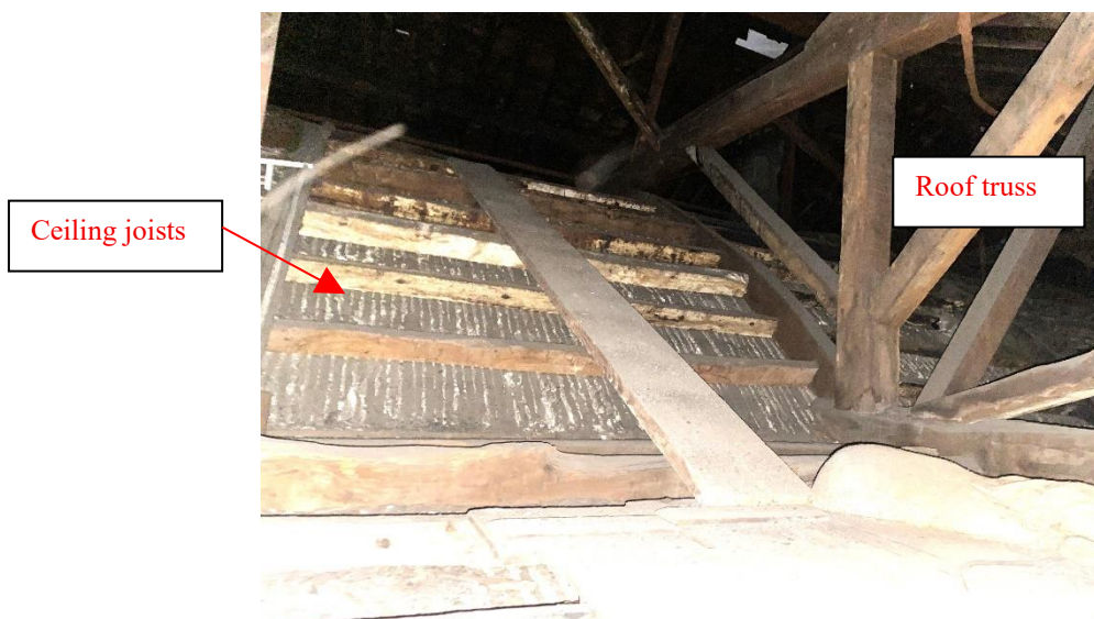
Figure 5. Ceiling construction from within roof void.
