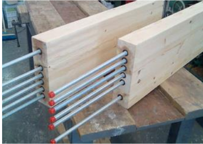
Figure 15. Epoxy resin timber beam repair.
