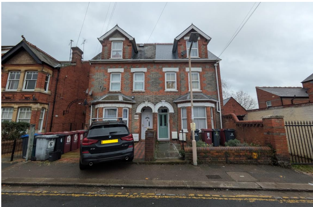
Figure 1 Site photo taken by case officer on 9 January 2025. No. 4 Prospect St to the right.
