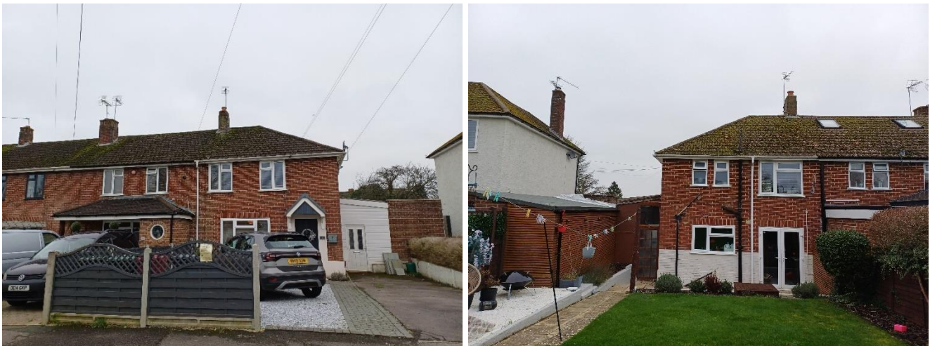
Fig 1: Views from the front and rear of 66 Mayfair, taken 23/12/2025
