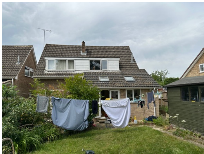
Photos – Existing Front & Rear Elevations
