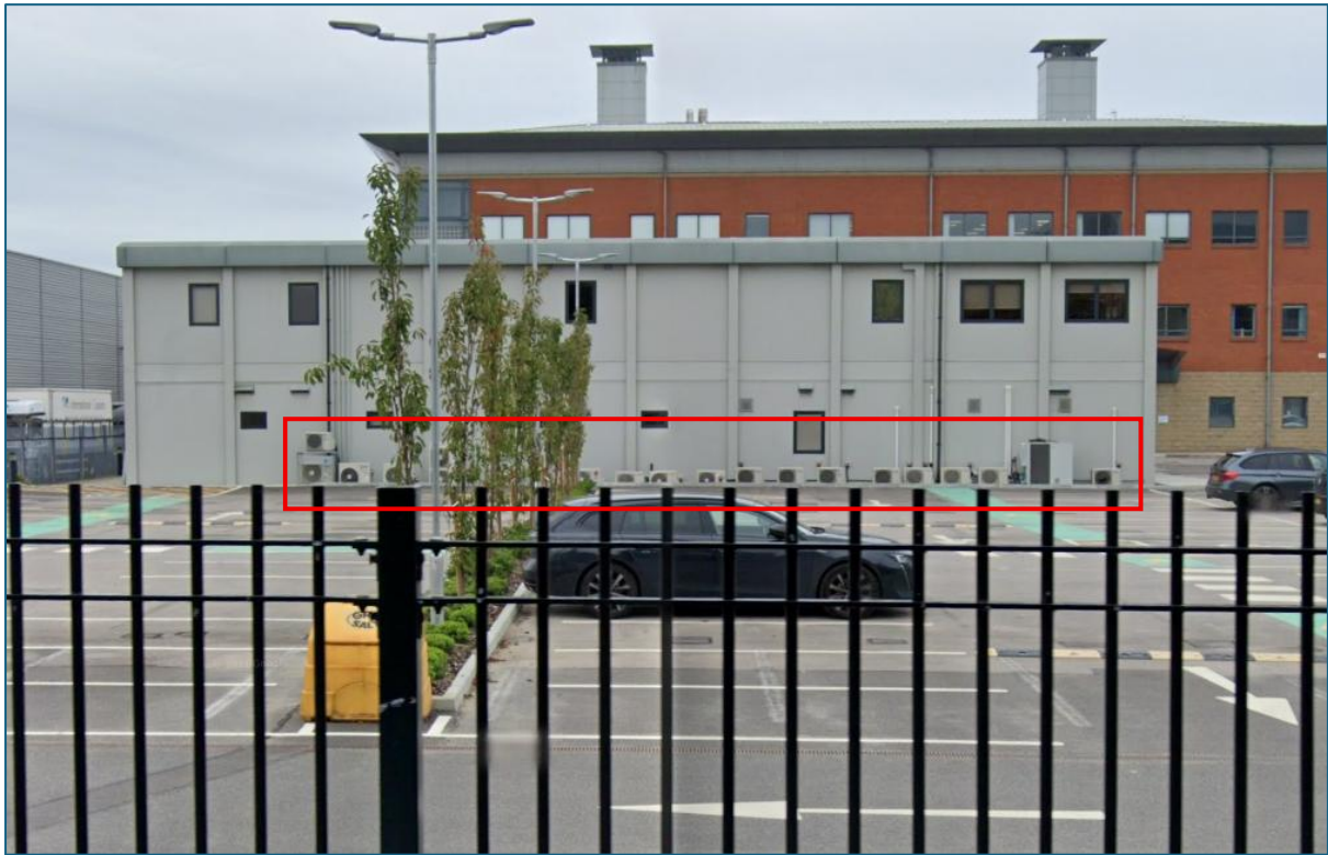
Previous AC Condensers (October 2020)
