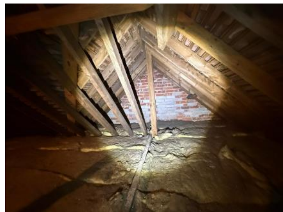
Photograph 14. Internal face of northeast gable
