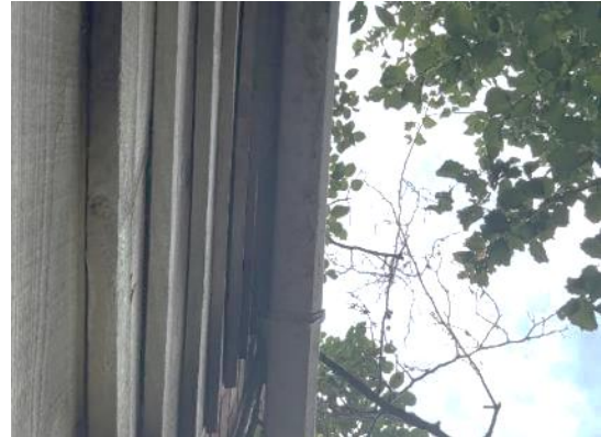
Photograph 20. Close-up of lifted timber cladding
