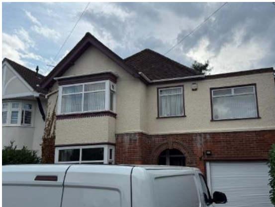
Photograph 1. East elevation of B1
