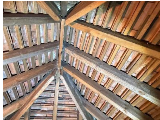
Photograph 12. Close up of B1 roof coverings
