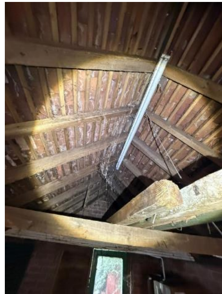
Photograph 24. Roof structure and underside of coverings
