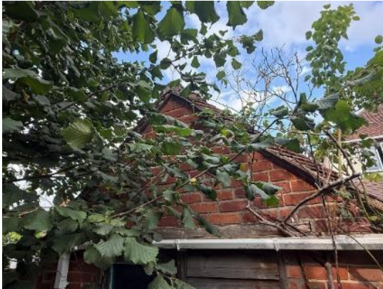
Photograph 19. Southwest elevation of B2
