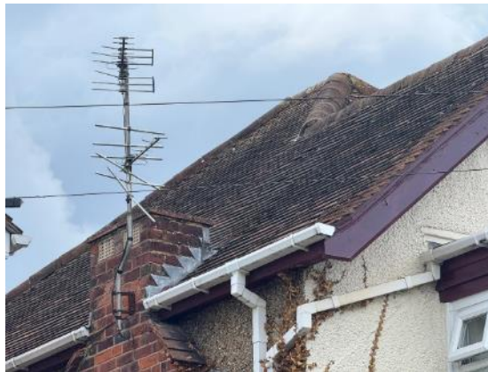
Photograph 4. Southeast elevation roof
