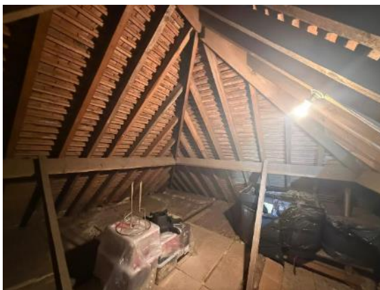
Photograph 13. B1 roof void with water tanks
