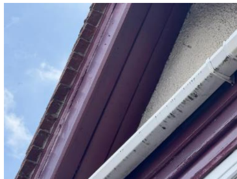
Photograph 3. Soffit gap
