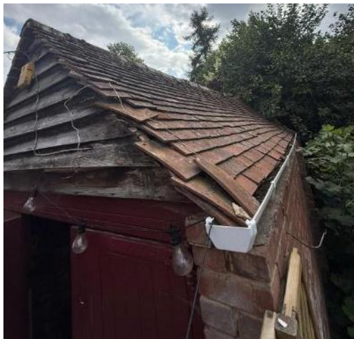
Photograph 22. Southwest elevation of B2
