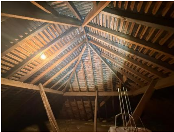
Photograph 11. Roof void of B1
