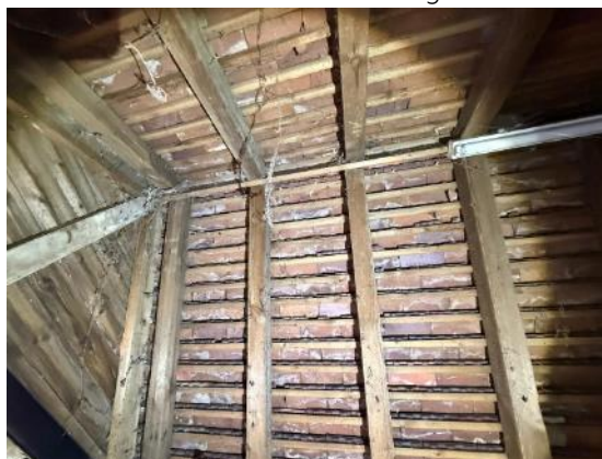
Photograph 25. Underside of coverings and internal face of exposed timber cladding.
