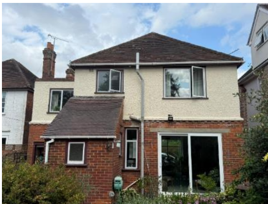
Photograph 5. Southwest elevation of B1
