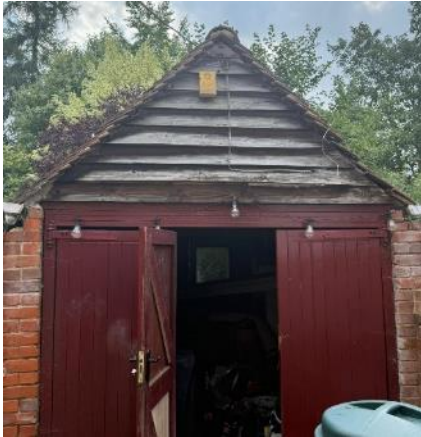
Photograph 15. Northeast elevation of B2
