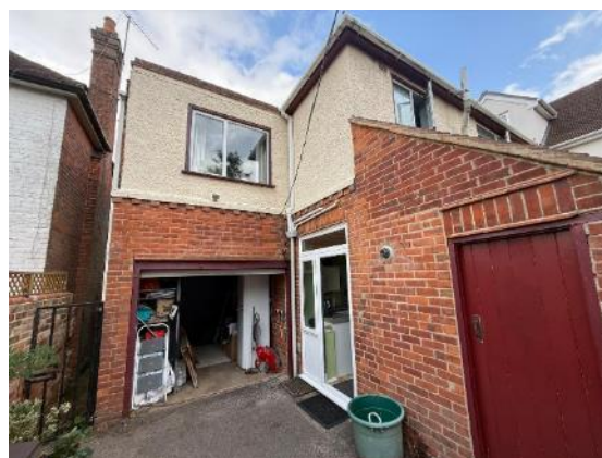
Photograph 10. Northwest elevation (wide angle)
