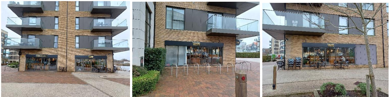
Figures 1 - 3: Views from the southeast (L), northeast (M) and northwest (R) of the property (12/01/26)
