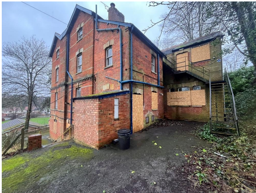
Plate 7: Northern double gabled elevation and rear elevation showing later extension
