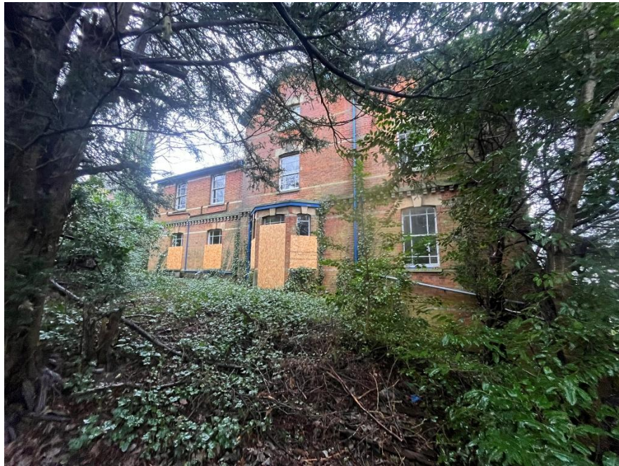
Plate 8: Western side elevation showing canted bay window and later two storey extension
