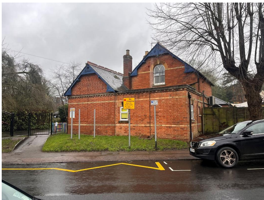
Plate 10: Different phases of construction on the lodge
