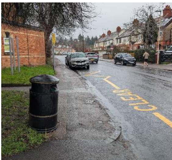
Photograph 2: Existing Hemdean Road Conditions looking north
