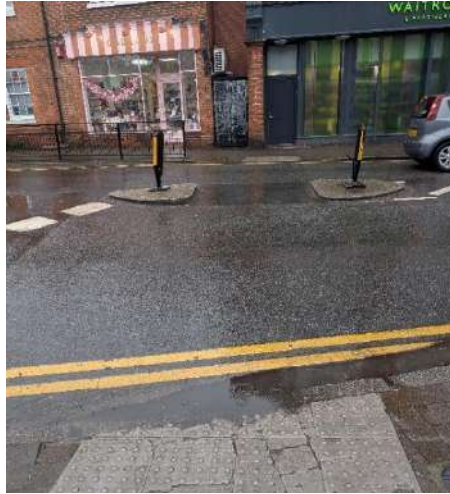
Photograph 5: Double Mini-Roundabout Refuge Island
