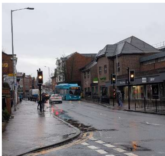
Photograph 4: Church Street Signalised Crossing
