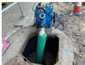
DRAIN LINING REPAIRS
