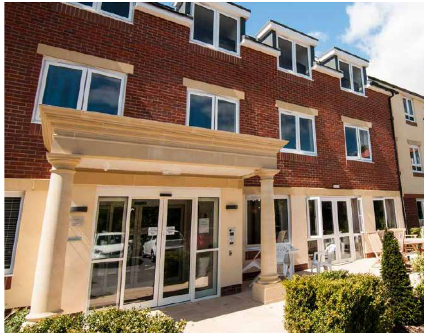
Secure Main Entrance from Parking
