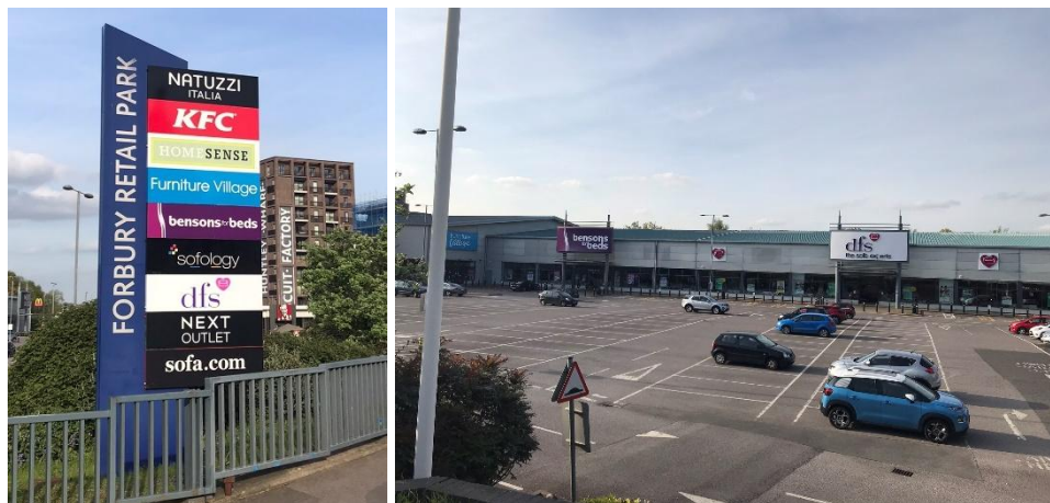
Entrance sign (left) and retail units with car park in the foreground (right)
