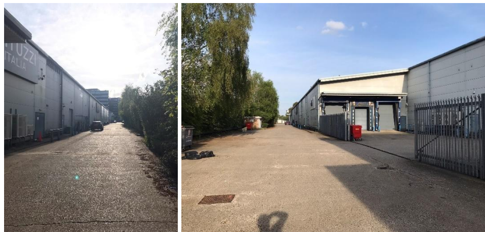
Rear loading bays
