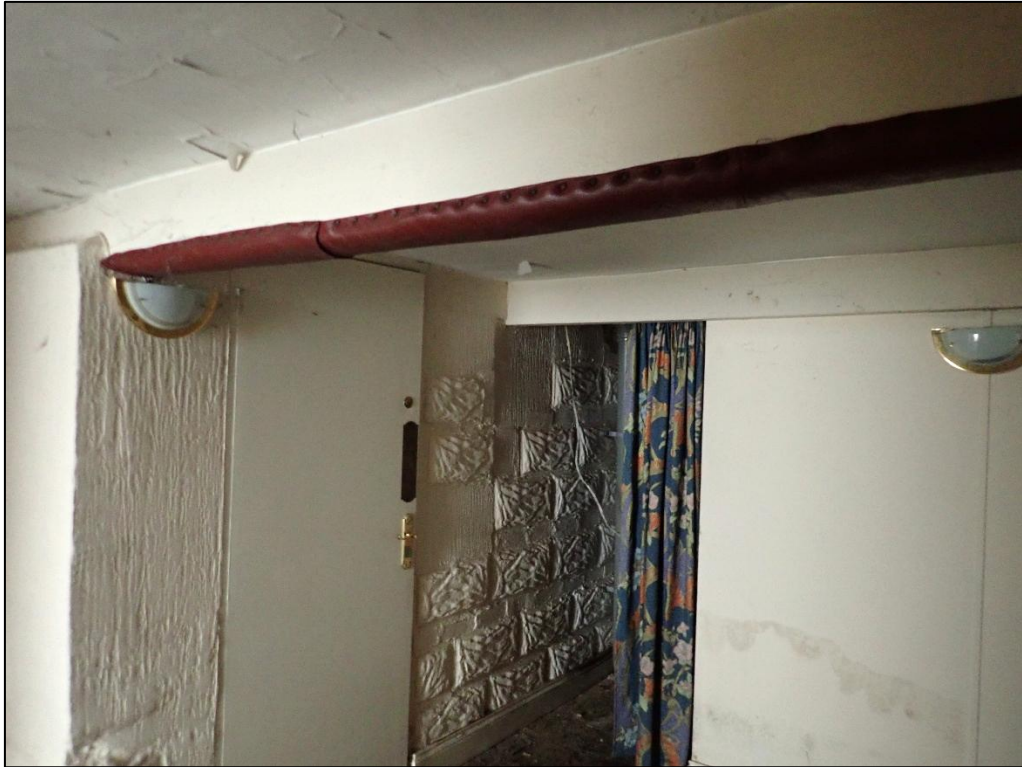
Figure 9. Partial view of the partitions within the basement, with the two downstand beams running left-to-right.
