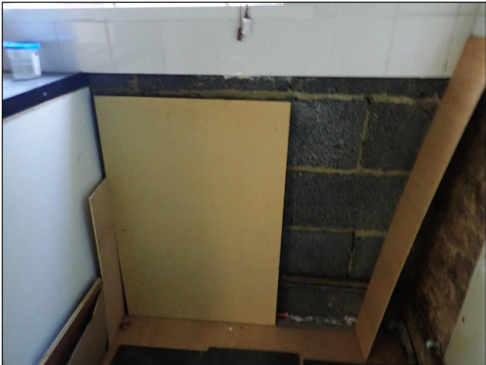
Figure 17. View of the exposed blockwork in the existing kitchen.
