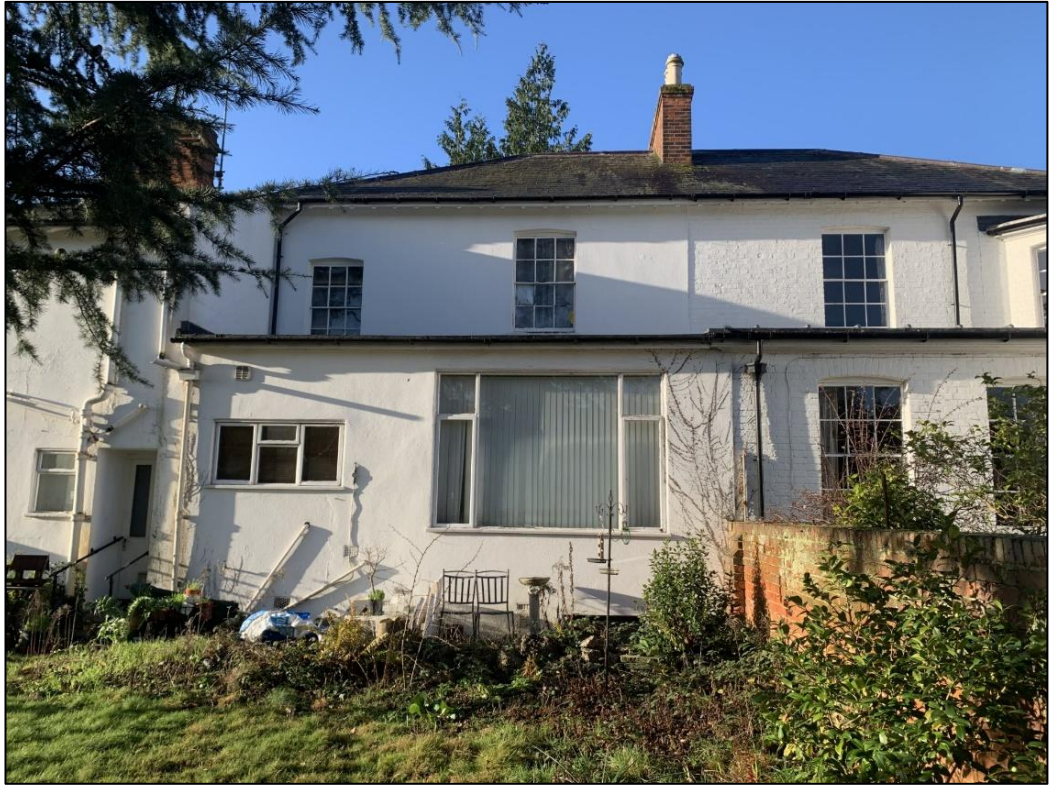
Figure 16. View of the rear elevation of the existing single-storey, rear extension, with No. 39 on the right-hand side.
