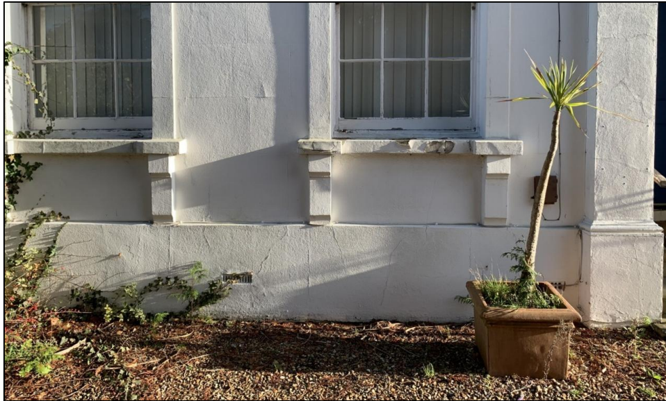
Figure 10. Current view beneath the ground-floor windows, where the lightwells will be located.
