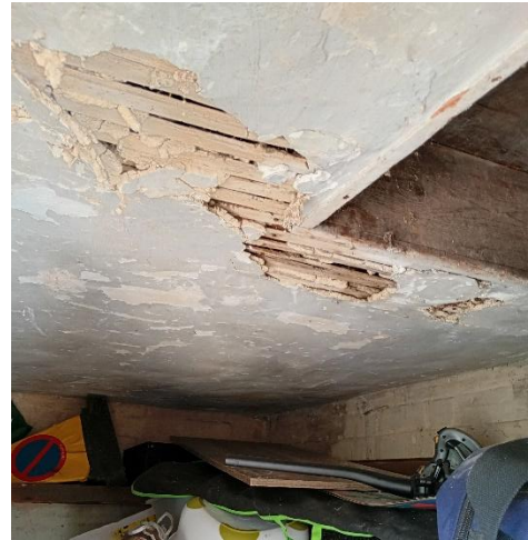
Figure 5: The hatch in the former stables and the condition of the lath and plaster
