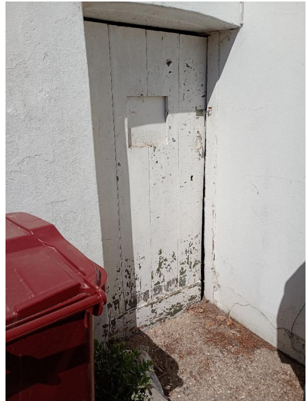
Figure 5: The hatch in the former stables and the condition of the lath and plaster
