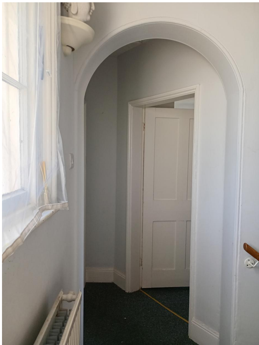
Figure 12: The angled wall behind the archway to be reconfigured
