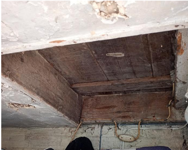
Figure 5: The hatch in the former stables and the condition of the lath and plaster
