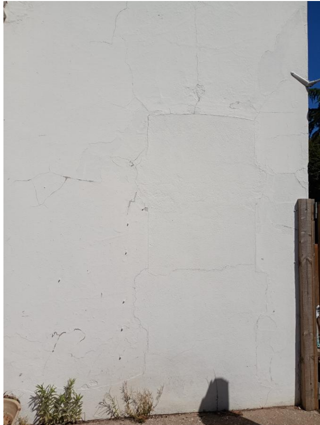
Figure 7: The outline of the former window opening
