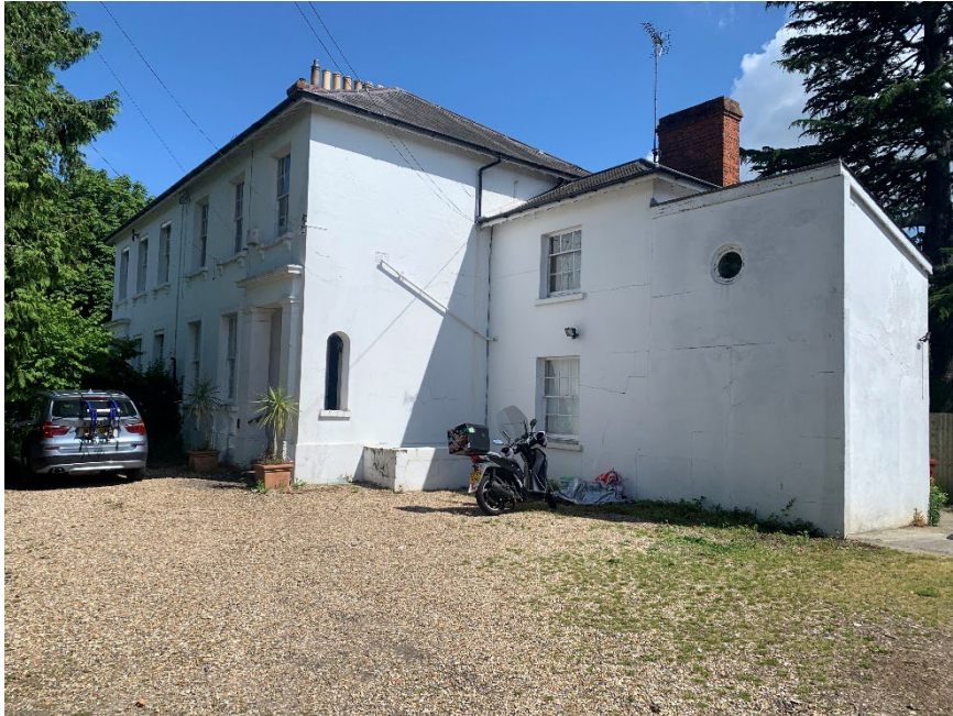
Fig 2. Photo of 41 Eastern Avenue from the South looking at the front of the property
