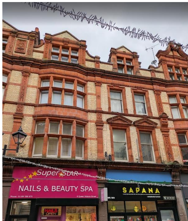
Figure 1 Upper floors at the front of 8 Queen Victoria Street. Image taken by case officer on 8 December 2025.
