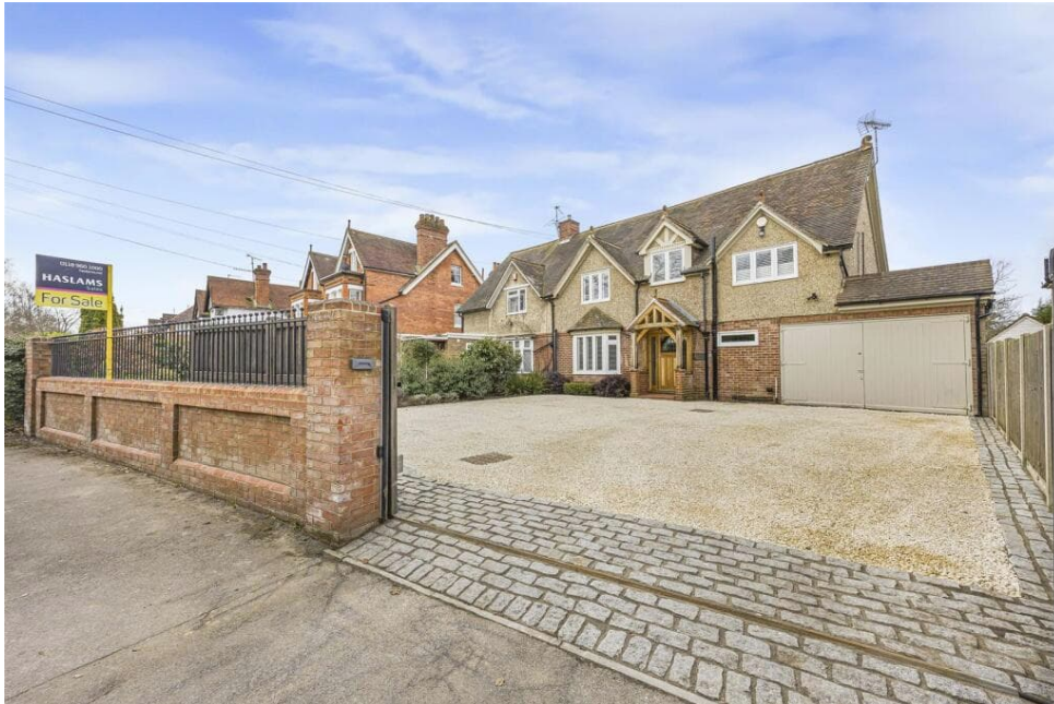
Existing front elevation showing the existing porch, this also show the ample size of front garden and drive
