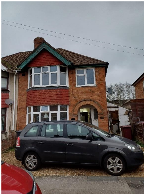
Fig 1: View from front of 180 Liverpool Road, taken 23/12/2025
