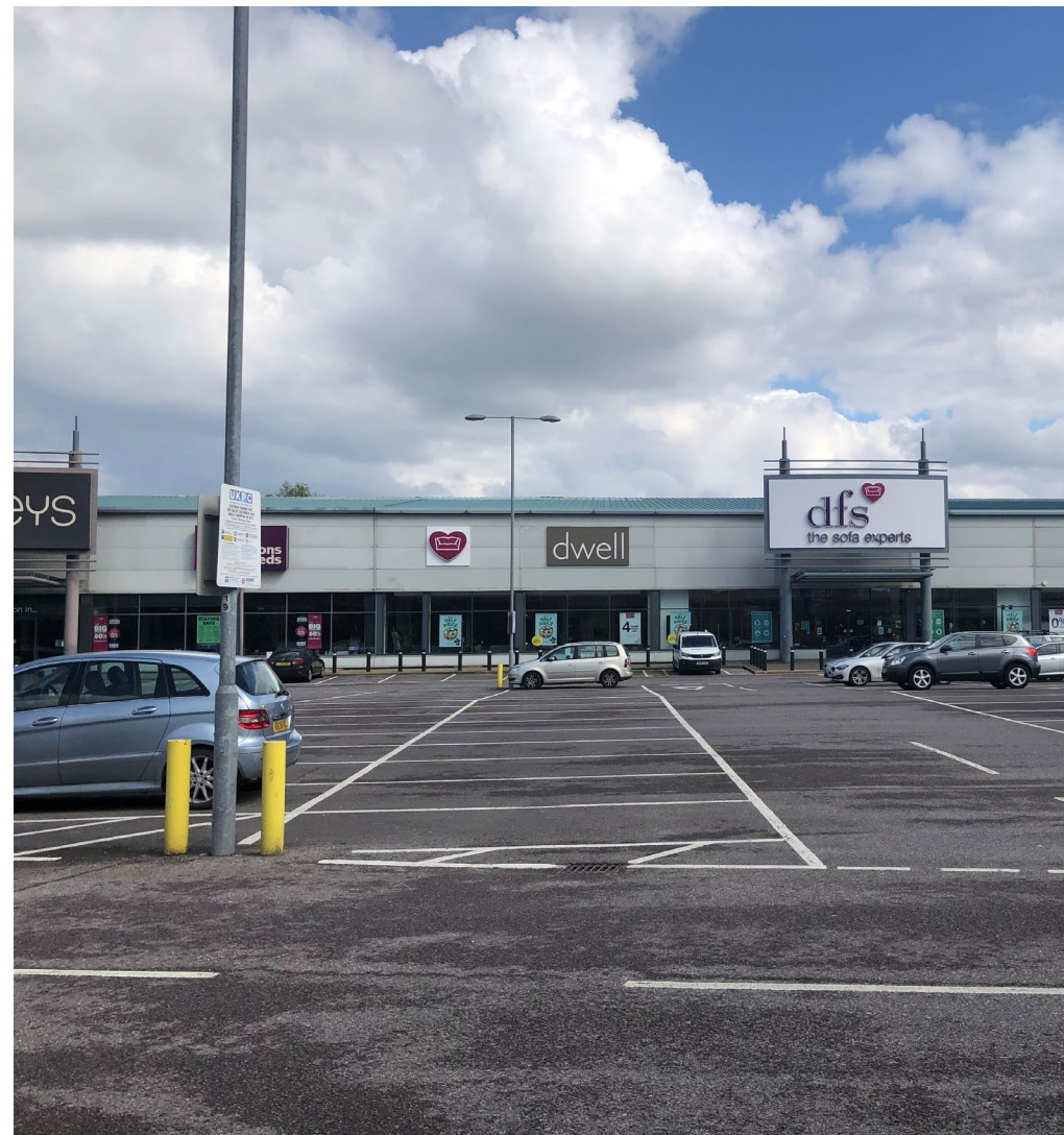
2. Forbury Retail Park - view towards existing building
