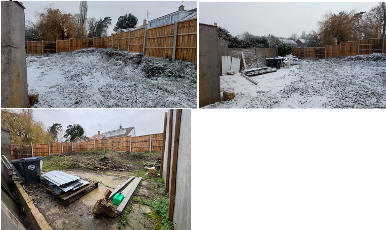
Fig 8 Sub divided land to rear of 5 Stoneham Close
