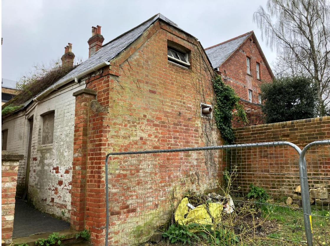
The rear of the garage
