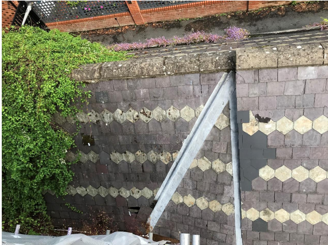
View of the roof
