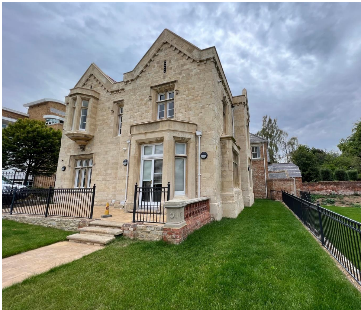
The refurbished no 17, now a staff wellbeing centre
