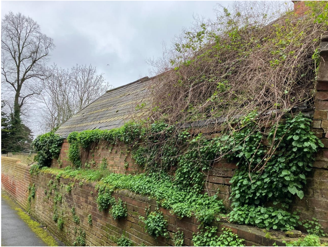
The north elevation showing the boundary wall to number 15 and the general foliage surrounding the building
