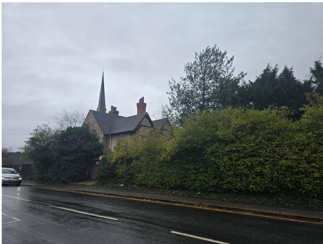
Photo 1 – View of 11 Glebe Road from the public highway
