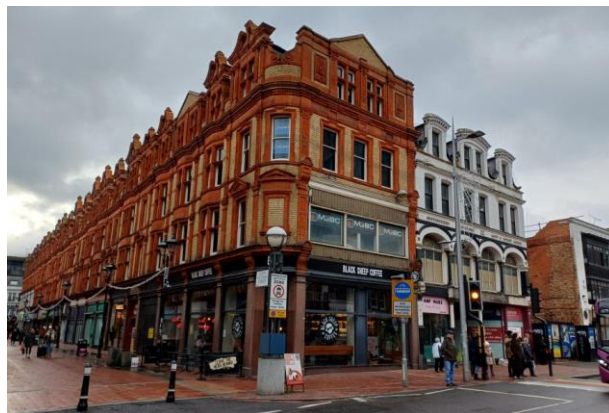
The application site looking south from the junction of Station Road, Friar Street and Queen Victoria Street (09/01/2026)
