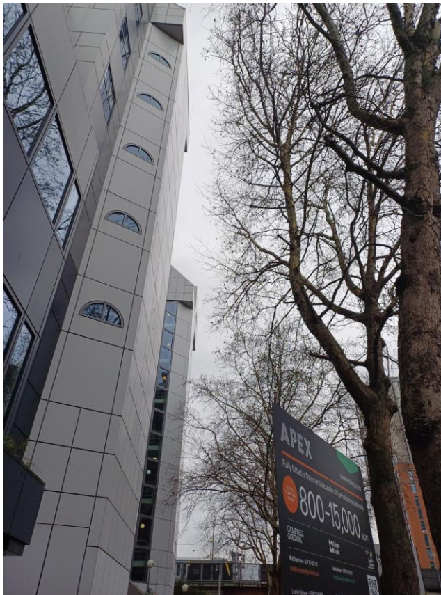
Figure 1: showing existing clearance
