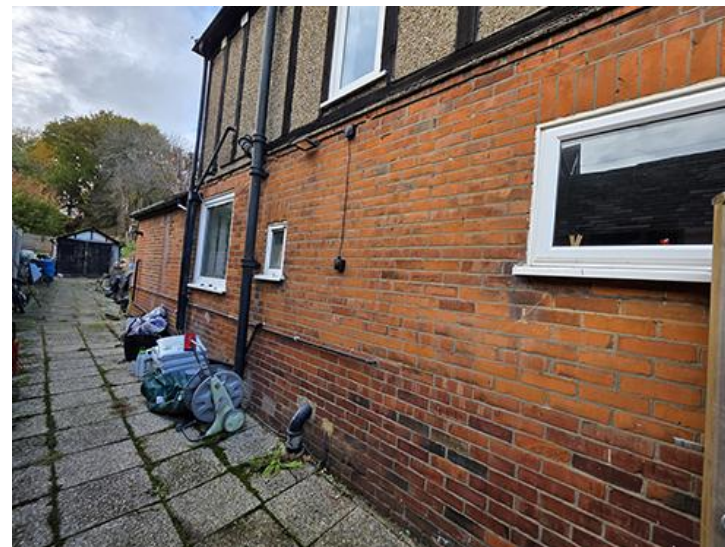
View of existing restricted side access
