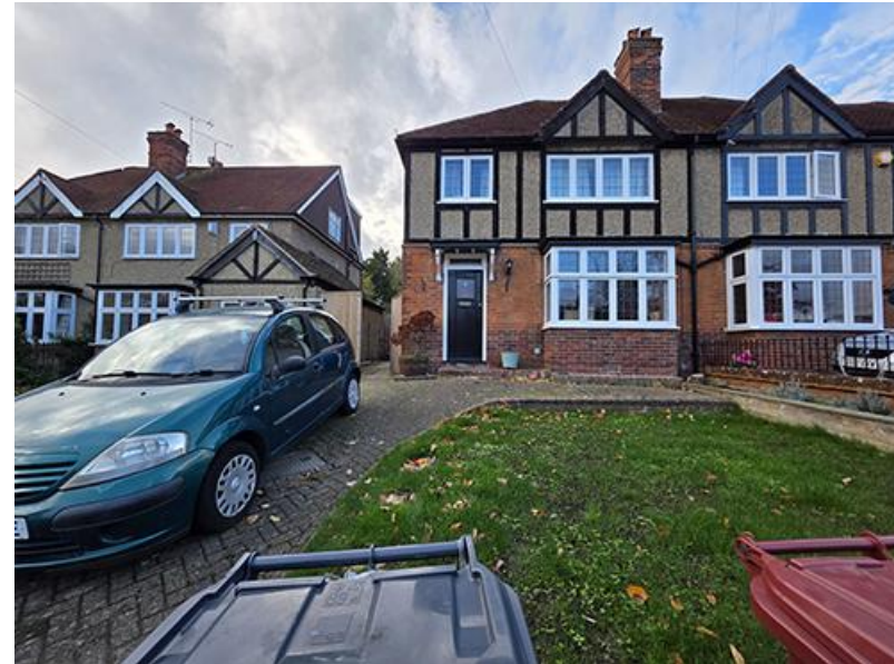
Existing dwelling frontage
