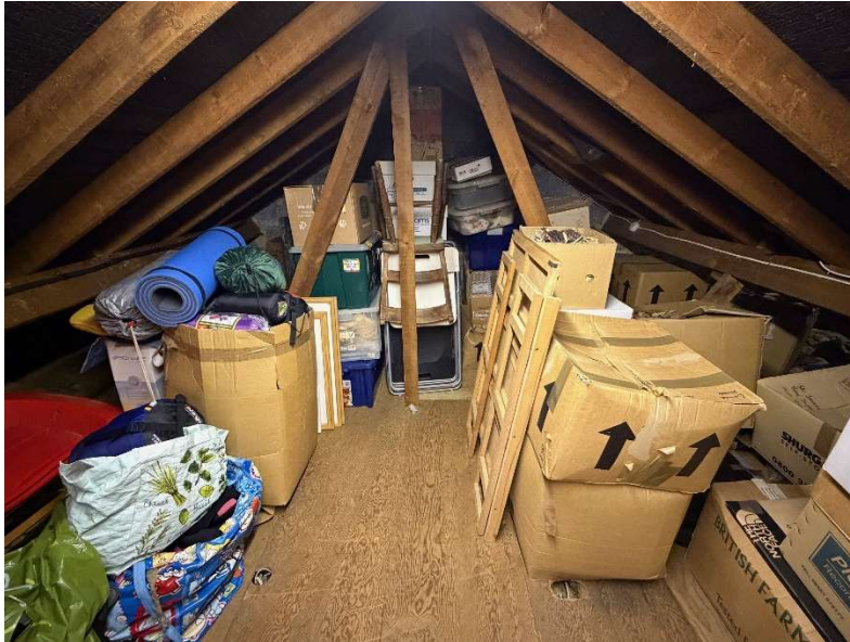
Photograph 12 – Eaves facing north
