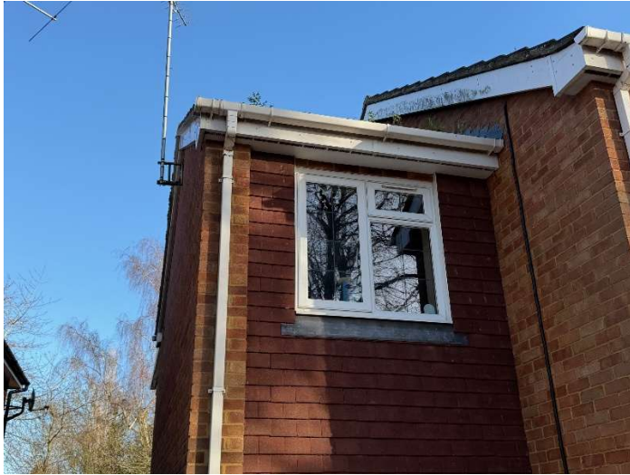
Photograph 2 – (Noth) West Elevation
