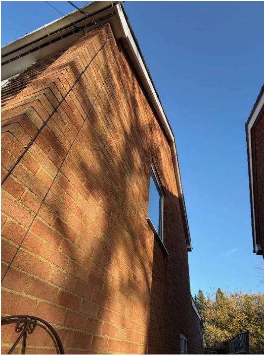
Photographs 4 and 5 – South Elevation
