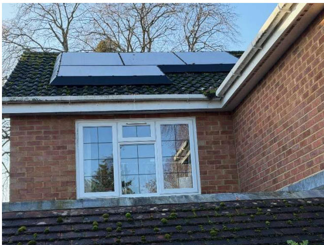
Photographs 8 and 9 – (South) East Elevation
