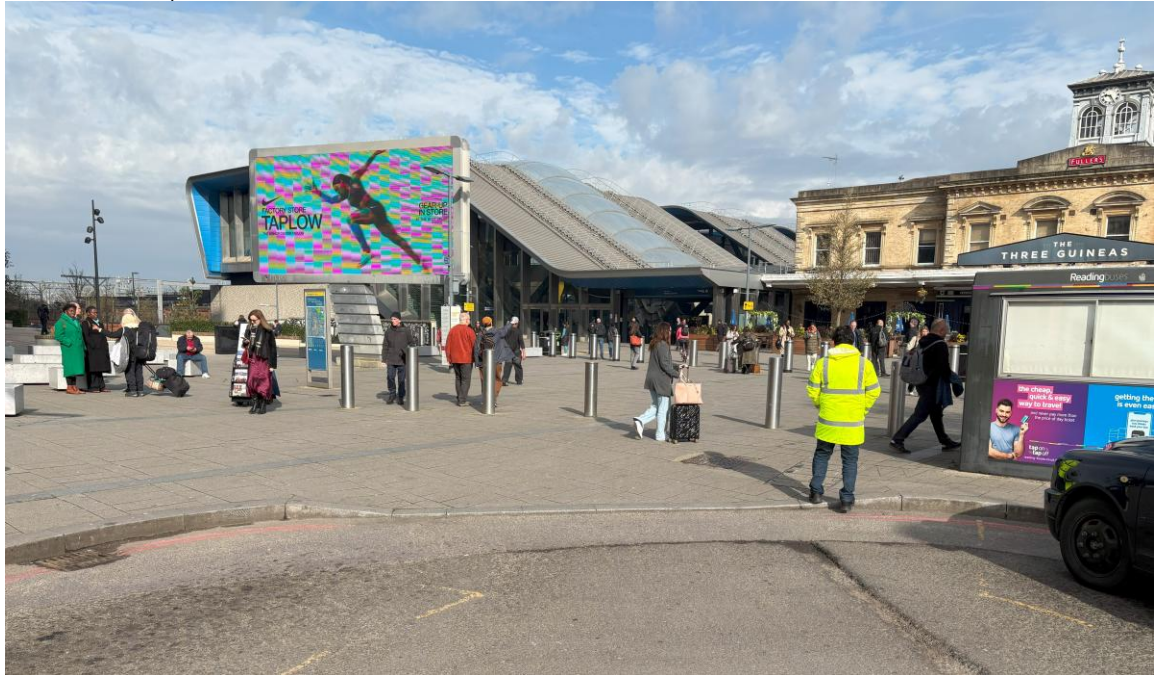
Photo 8: Station Square Entrance
