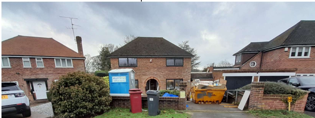
Front elevation and wider streetscene with replacement black window frames
