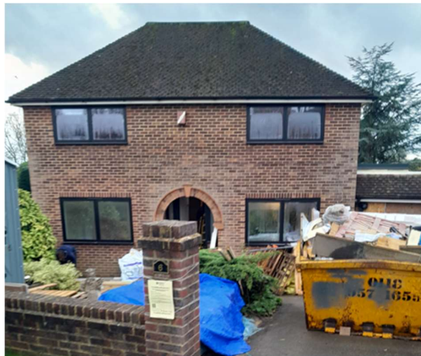
Front elevation with replacement black window frames
