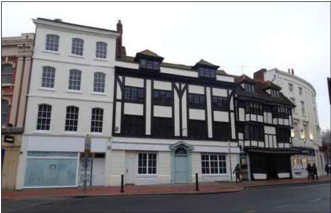
PHOTO: Elevation works in progress, making good to match existing finishes
