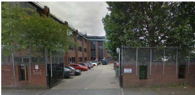
Fig. 05 Rear (Vehicular) Entrance
