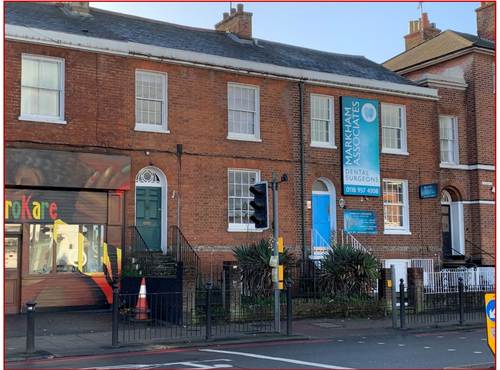
Plate 13 - Part of 149-169 Oxford Road viewed from the north side of Oxford Road
