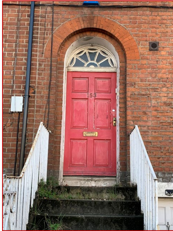
Plate 3 - Door entrance detail to 153 Oxford Road
