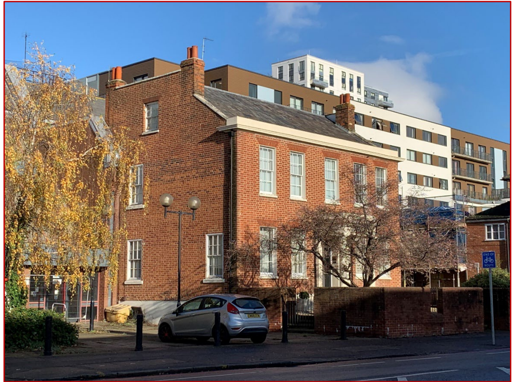
Plate 9 – Subject building from southwest in Conservation Area
