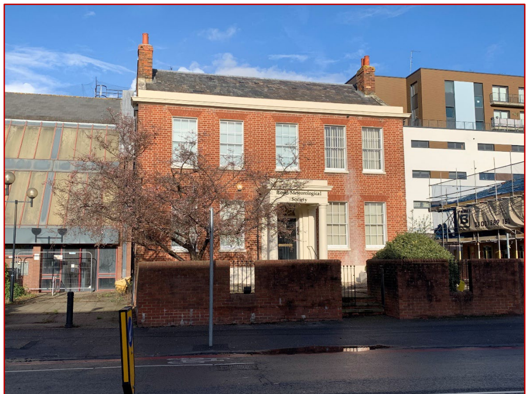
Plate 10 – South elevation subject building from Conservation Area
