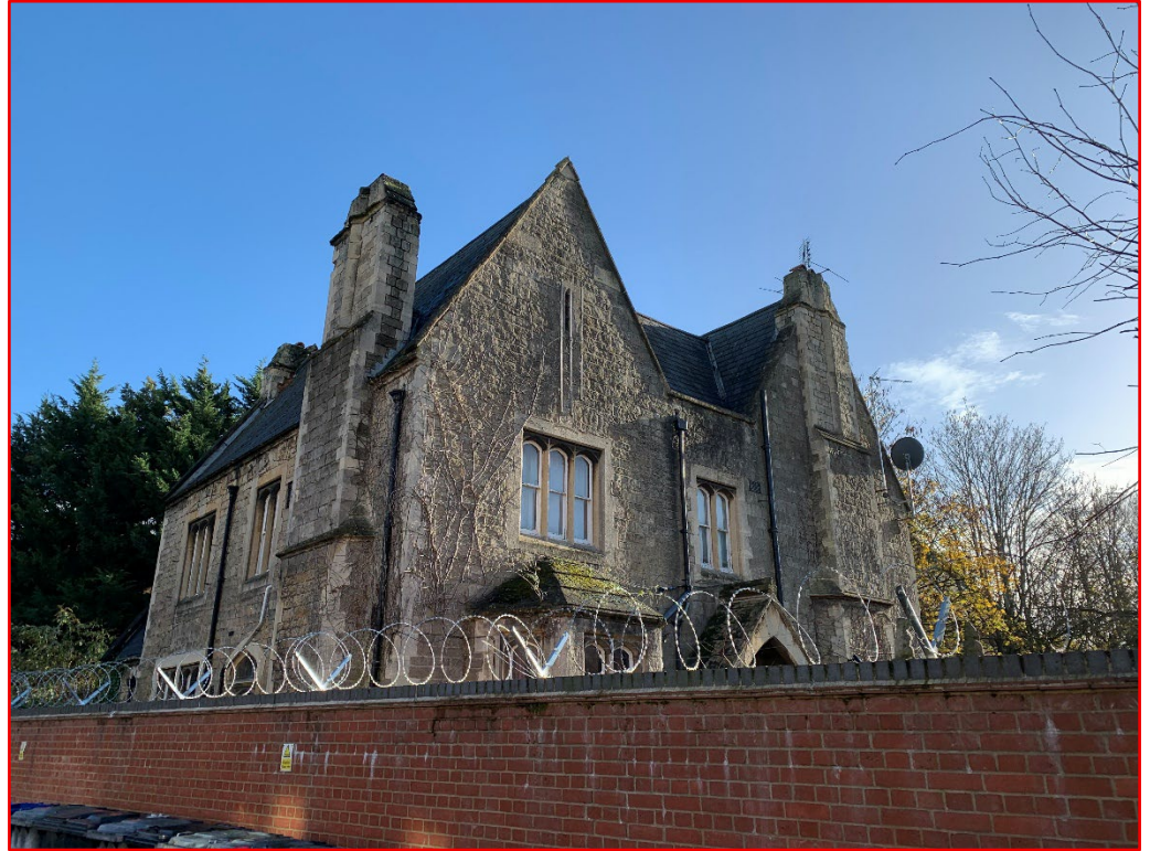
Plate 15 – 118 Oxford Road, viewed from the northwest
