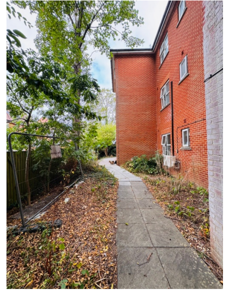
Facing north (from centre of site)
