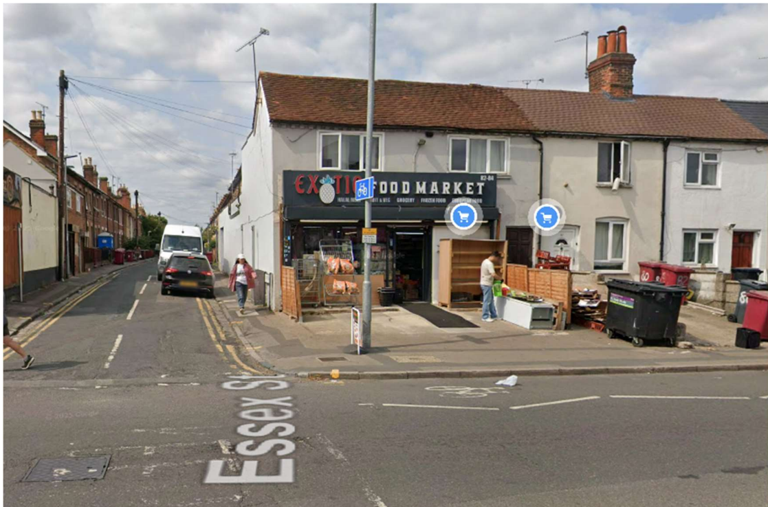
Existing front elevation (with unauthorised signboard)
