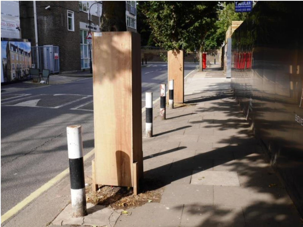
Photo 8: Example of stem box protection.
