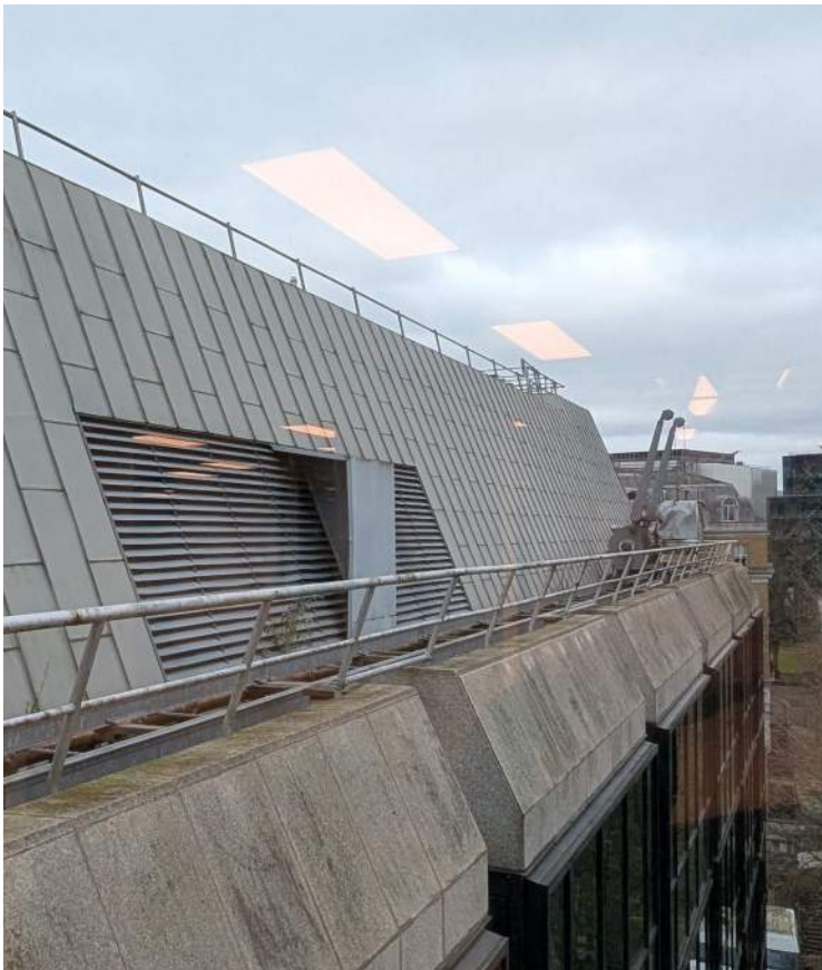
Ventilation grilles to existing mansard roof
