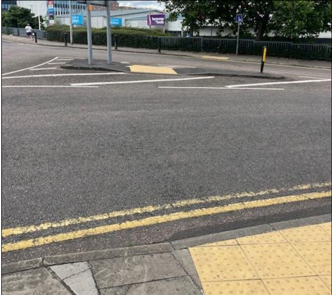
Figure 3.2: Kenavon Drive Crossing (with Tactile Paving)
