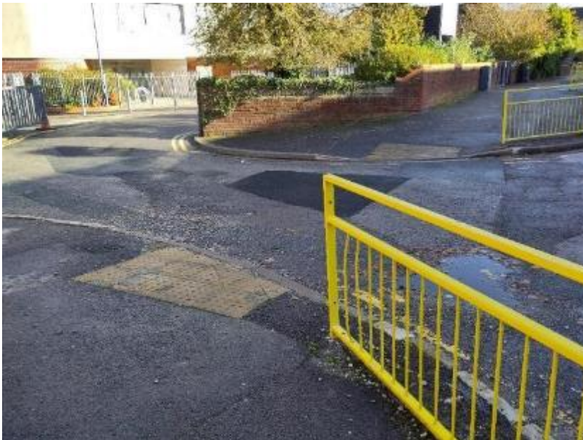
Informal Drop Kerb Crossing with Tactile Paving at St John's
