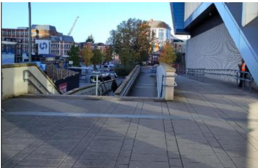
Ramp & Stairs to Reading Railway Station Underpass
