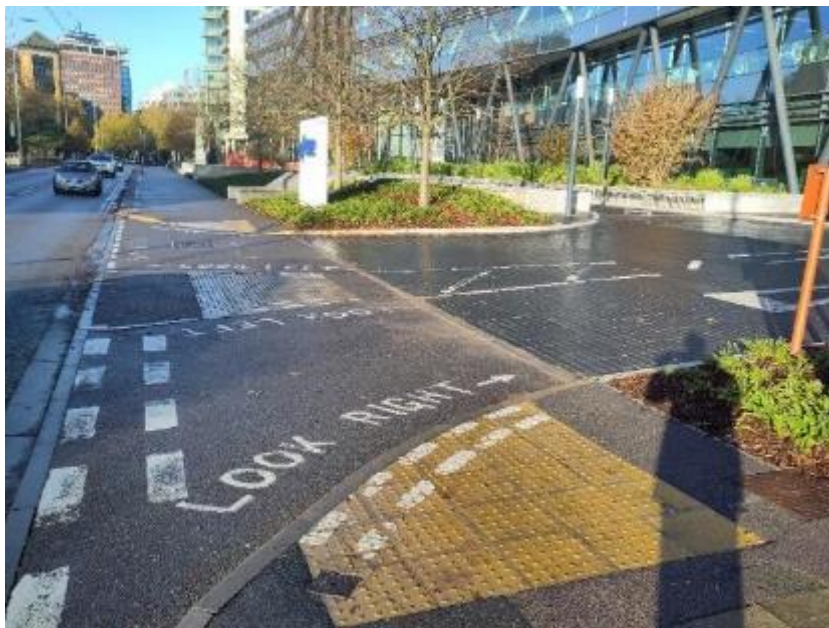
SWE Access Point Crossing
