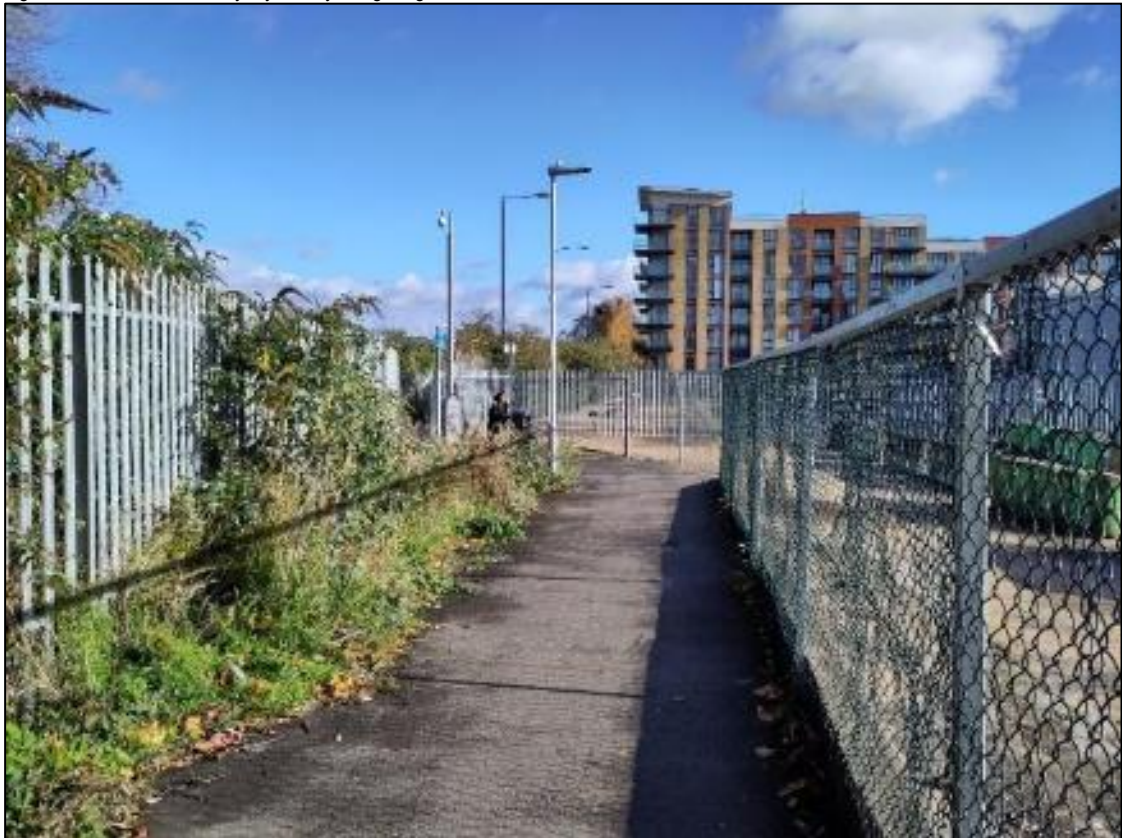
Figure 2.9: Shared Footway/Cycleway – Lighting and CCTV
