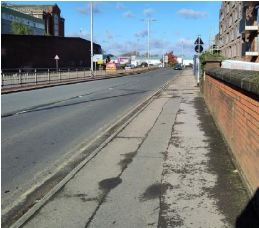
Forbury Road Footway
