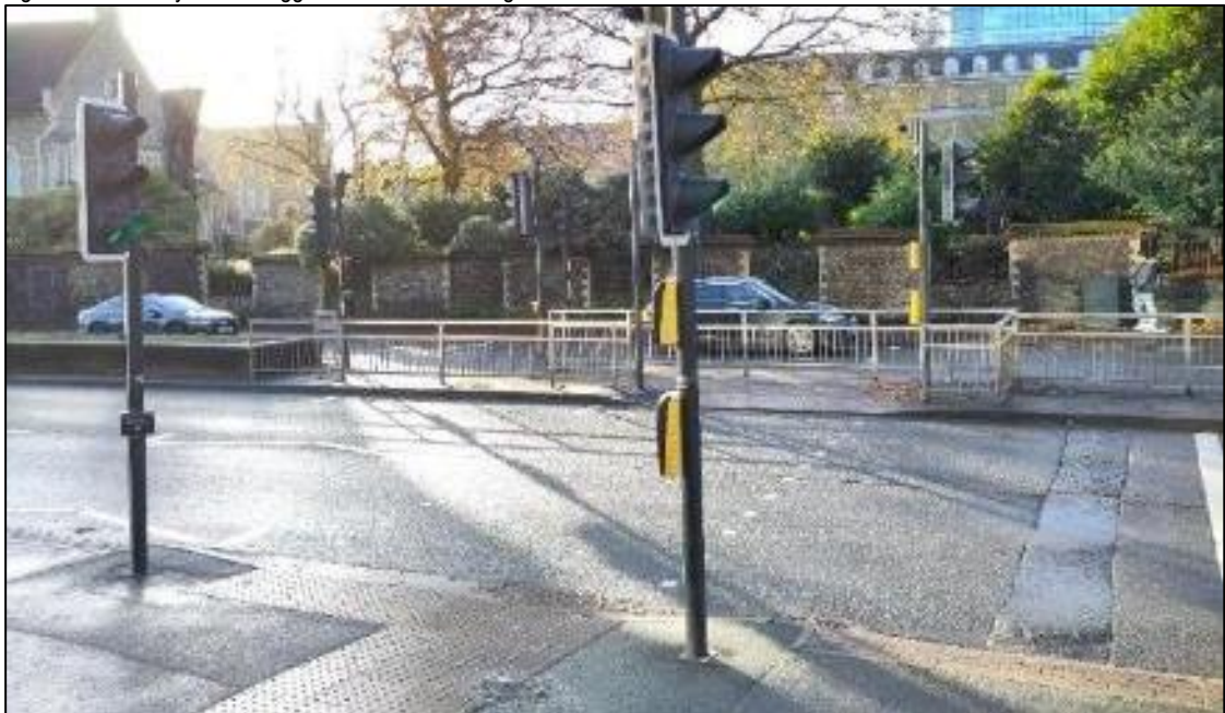
Figure 2.8: Forbury Road Staggered Pelican Crossing
