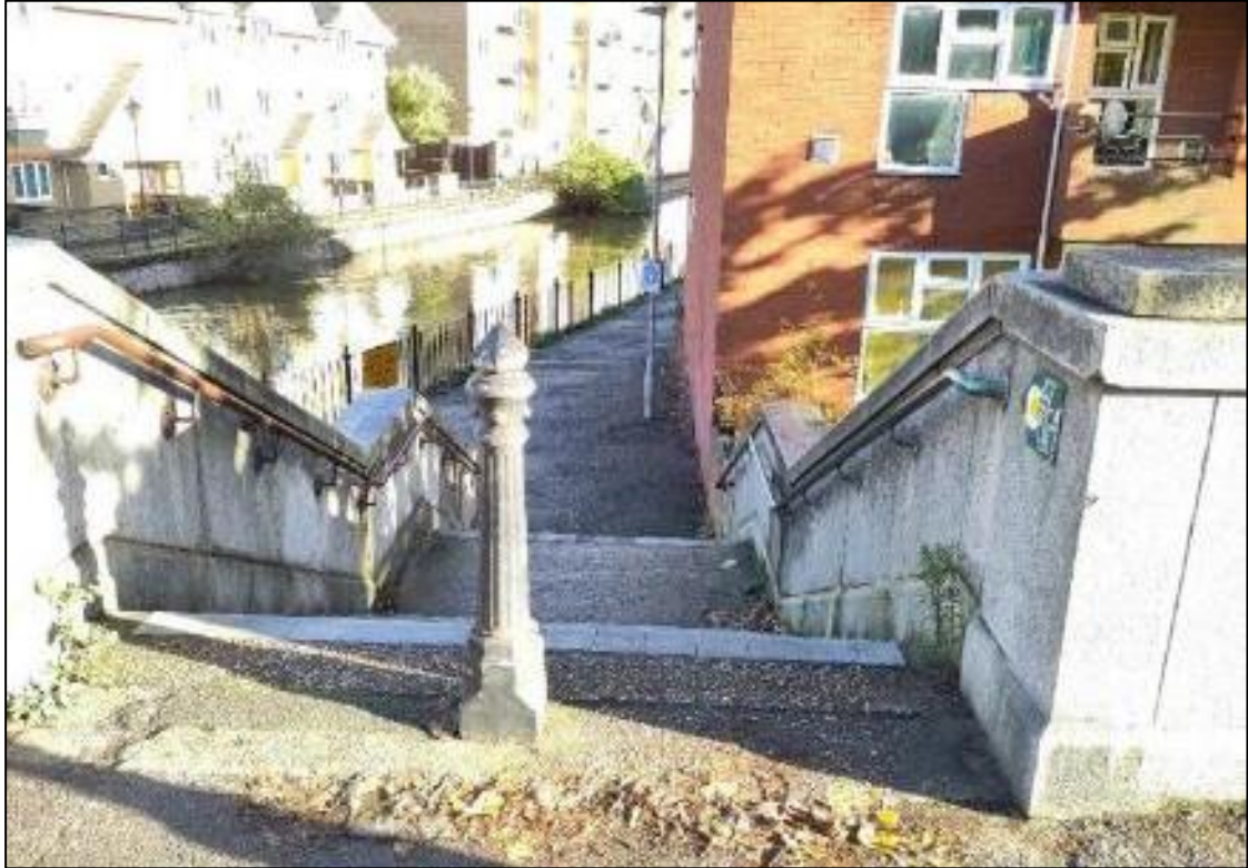
Figure 2.17: Stairs to River Kennet
