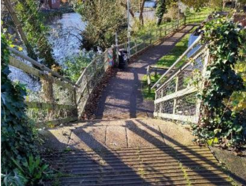
Stairs with Handrail to Bridge over the River Kennet
