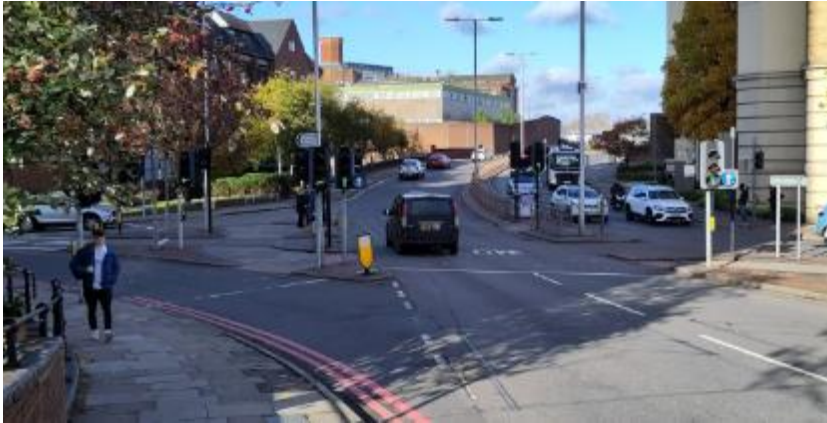
Forbury/Kings Road Crossings
