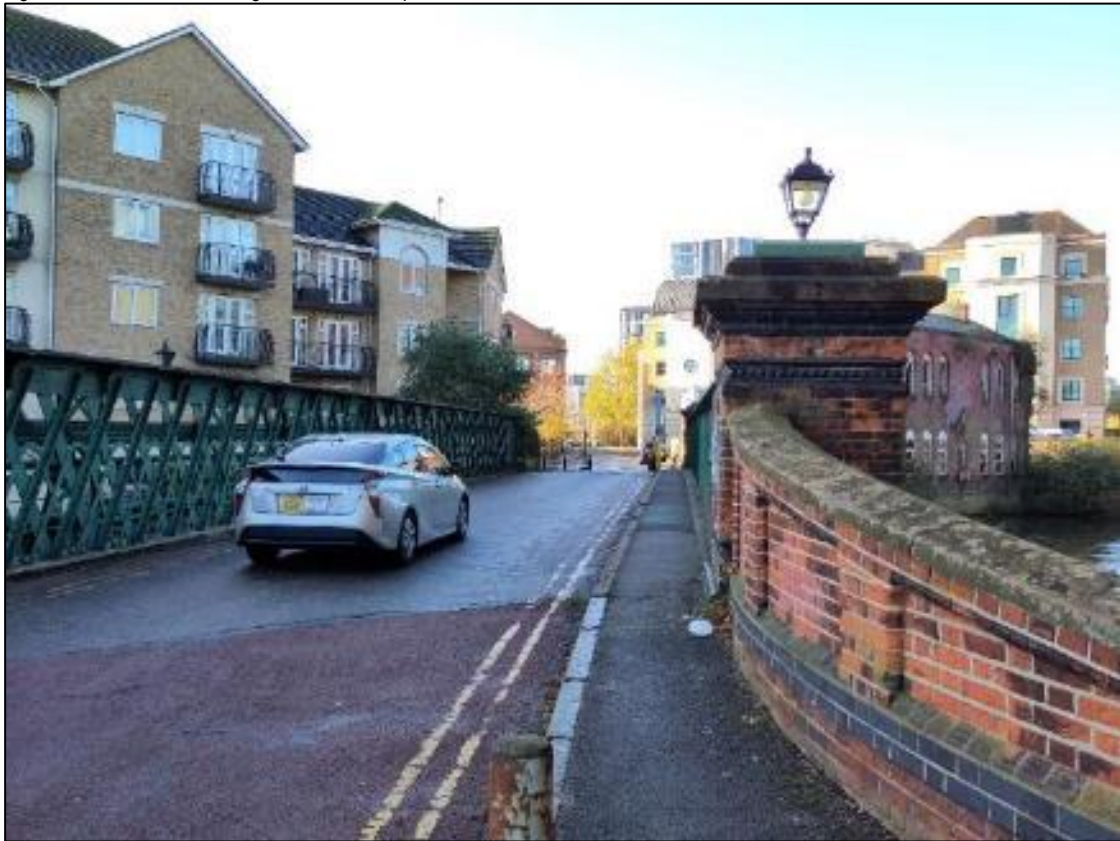
Figure 2.16: Gas Works Bridge – Narrow Footpath and Bollards
