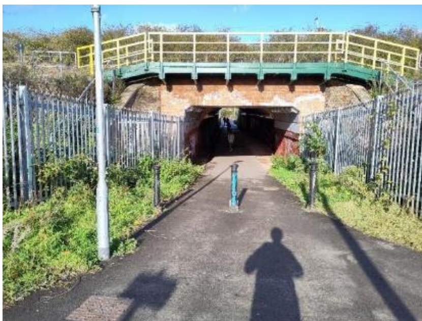
Biscuit Tunnel – Lighting
