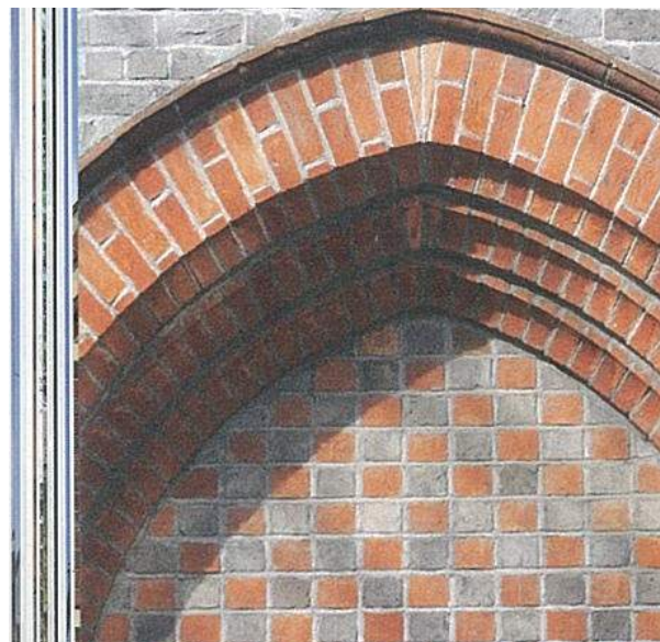
Voussoir Arch with Red and Grey Chequerwork
