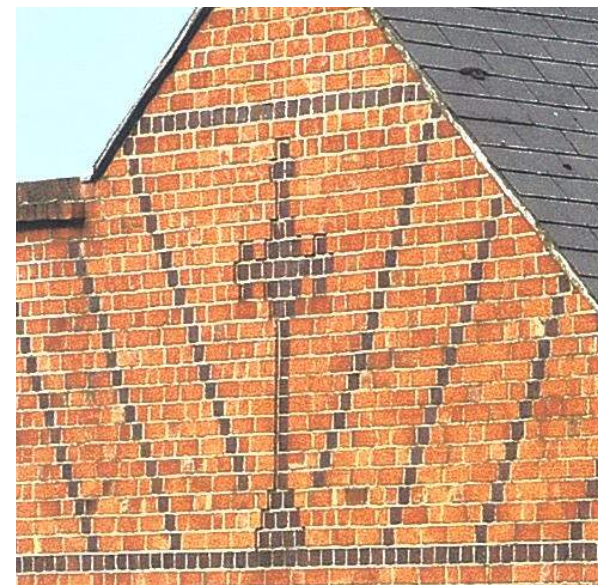
Stepped Crosses of Purple Bricks, River Rd
