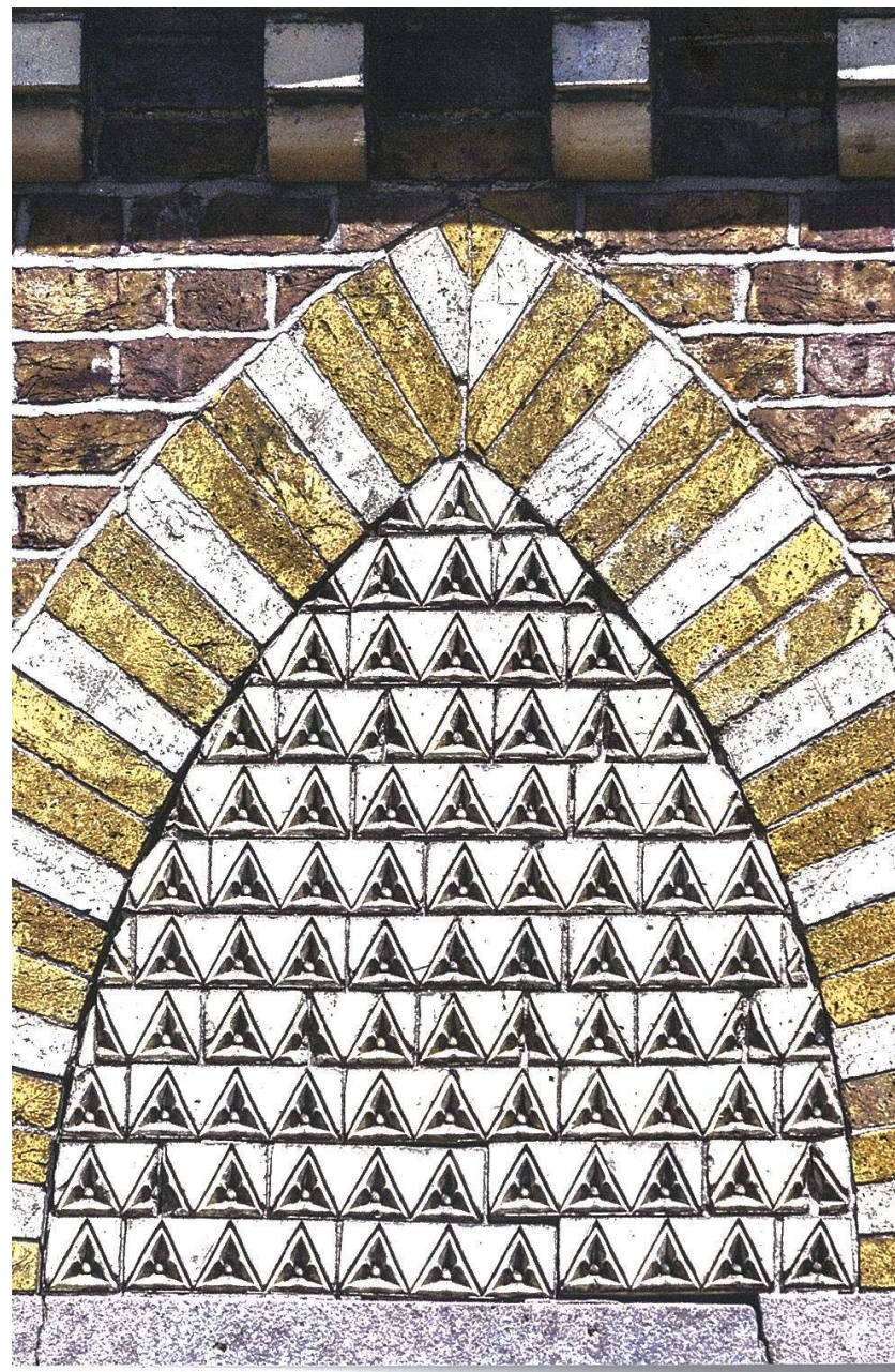
Decorative Brickwork on Christchurch Road
