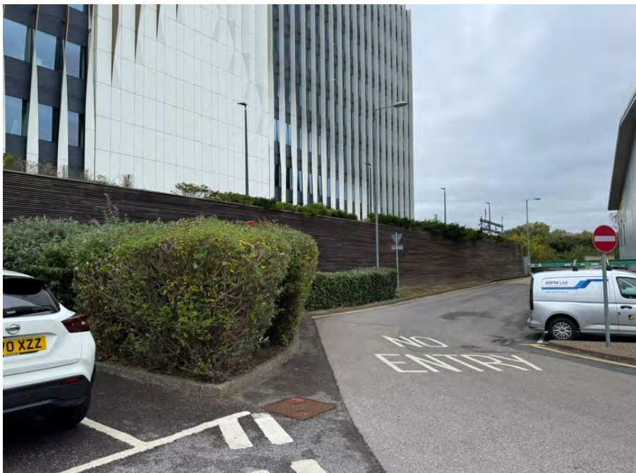
Photograph 2: Building and hardstanding (and wall) along western Site boundary.
