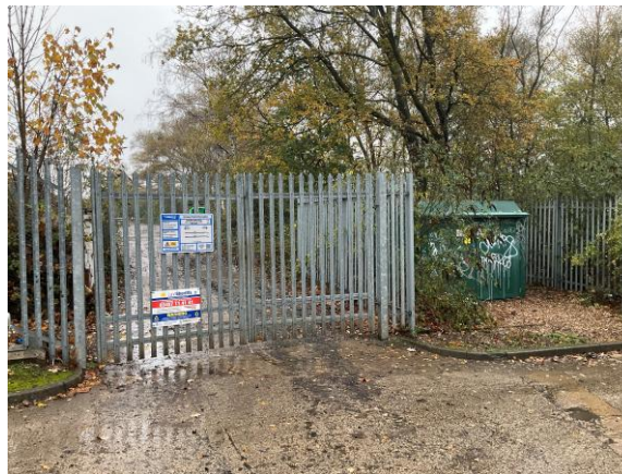
B5: Electrical substation and rail access in the north-east corner of the site.
