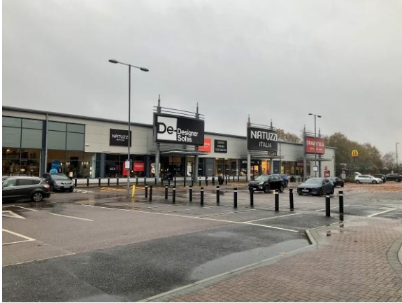
B1: General view of property looking towards north-east.
