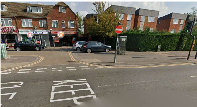
Existing streetscene looking east.
