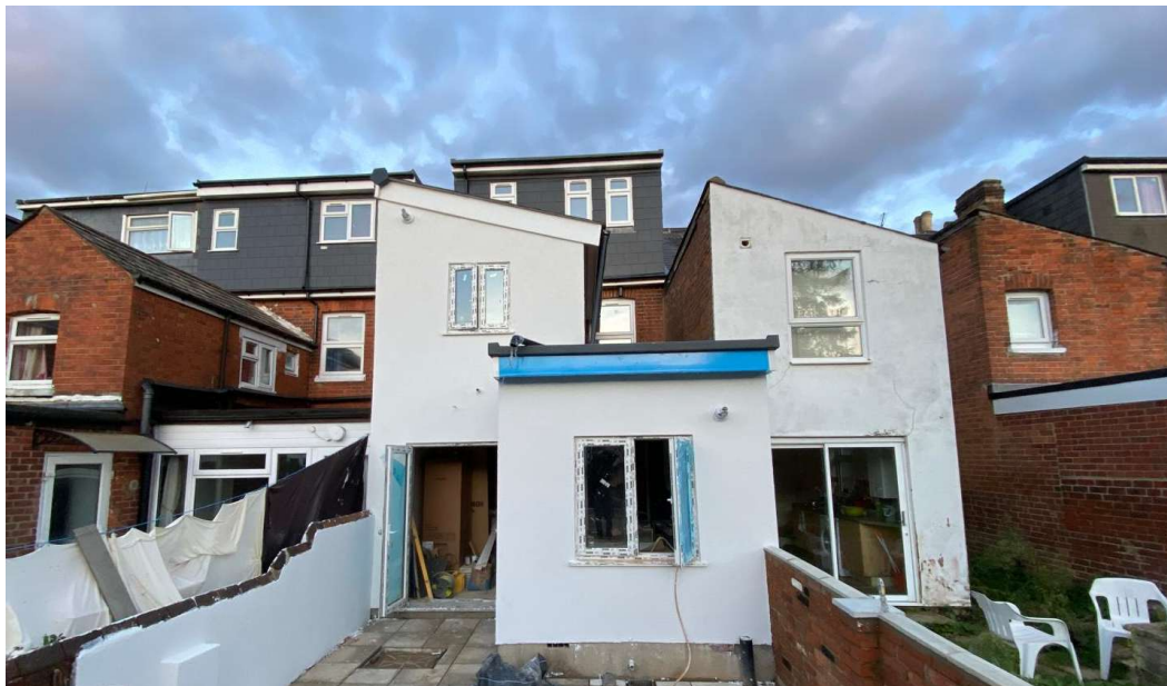
Figure 2: Photograph of rear of property (taken in 2022)
