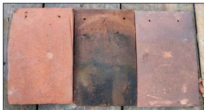
Reclaimed Roof Tiles
