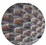
A1. dark brown brick with projecting brick detail.
