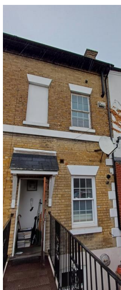
Location of the existing first floor flue
