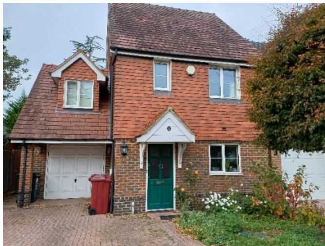
Fig 1: View from front of 2 Pantile Close, taken 17/10/2025
