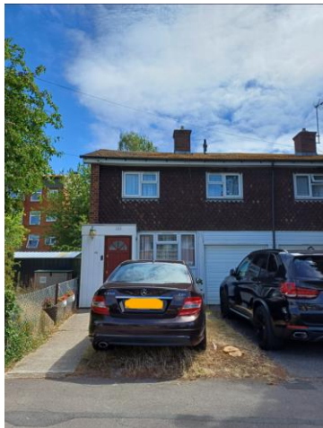
Fig 1: View from the front of 141 Appleford Road
